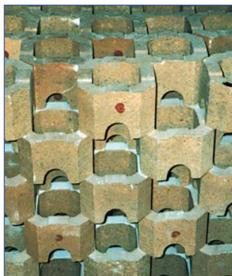
Typical regenerator chimney block packing during construction
