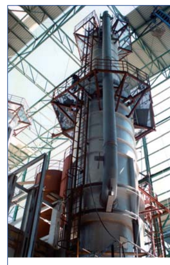
Tube cage recuperator
